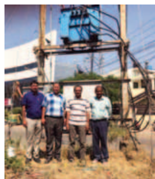
Figure 1. Metering on Proactive Repaired 200 kVA DT
